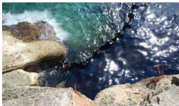
This photo, taken last October at Clifton Pier, shows oil seeping through a barrier presumably erected to contain it. The area suffers frequent spills and leaks of petroleum products and other toxic substances, most likely from one or more of the nearby industrial plants. However, in the absence of any official investigations by government, both the source of the leaks and the identity of the agencies that sporadically attempt to contain them, remains unclear.
