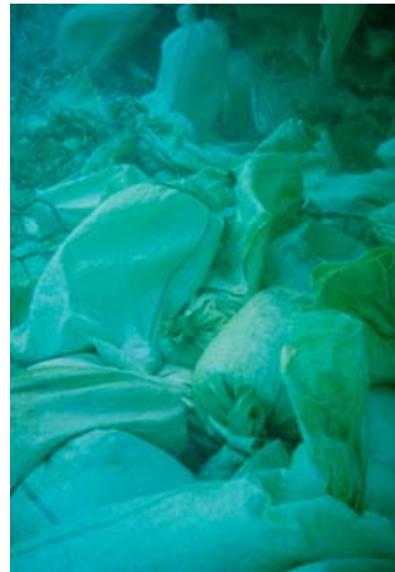
∨ ∨ ∨ Another 2002 photo which shows the polypropylene sand bags which are stabilizing the wire gabions.
