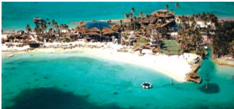
This 2002 aerial photo shows the long, thin, man-made underwater reef extending west from Simms Point/Nygaard Cay's Clifton Bay dock/jetty. The government alleged that Nygard "constructed groins, seawalls, berms, pylons and other underwater structures designed to act as dams capturing the sand."
